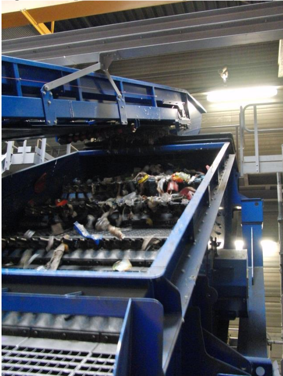
Figure 16: Dosing unit used to feed the NIR sorters
